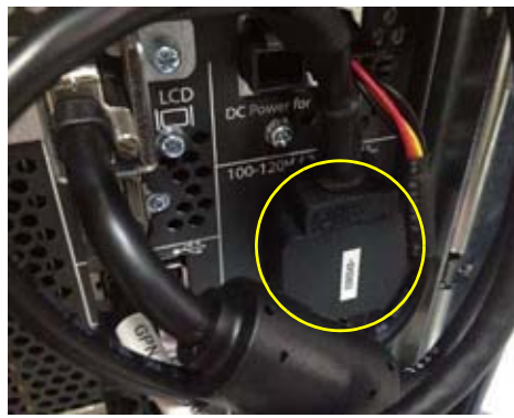
Inserting Printer Power cable into the Nest box
